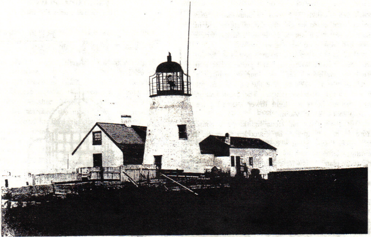
BIRD ISLAND LIGHTHOUSE Photograph taken before 1890
